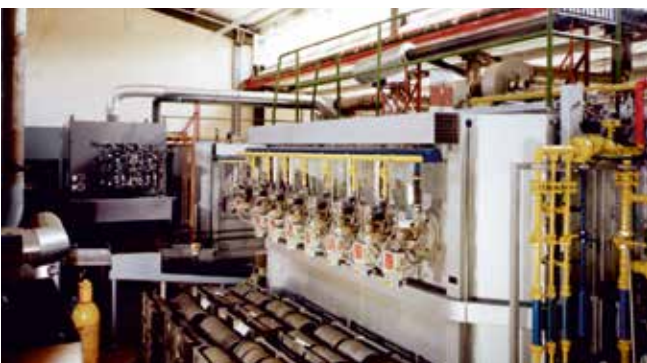
Rotary hearth furnace gas heated
